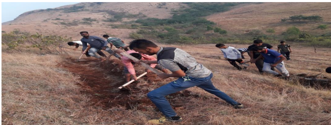
Volunteers digging Continuous Contour Trenches (CCT) on the hill at
