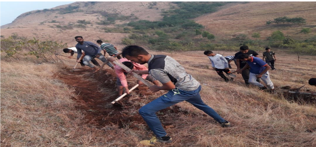
Volunteers digging Continuous Contour Trenches (CCT) on the hill at Dari
