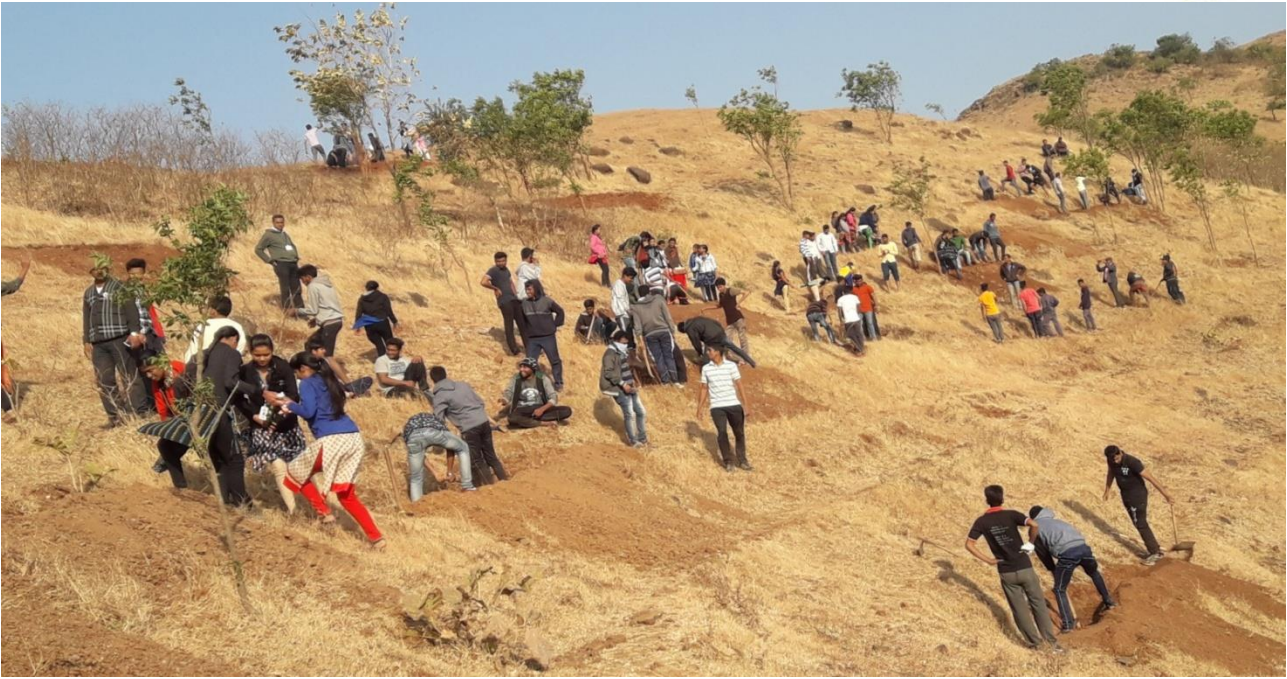
Volunteers digging Continuous Contour Trenches (CCT) on the hill at Dari
