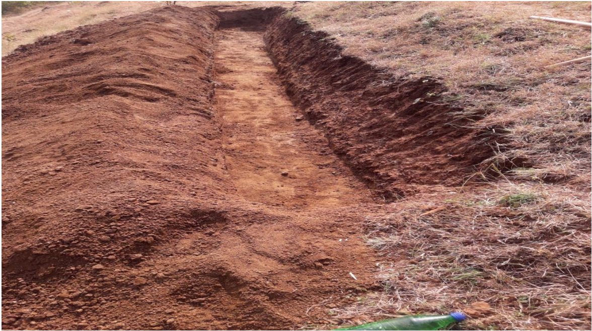
Volunteers dig a 15 * 2 * 2 length, width and depth CCT at the NSS camp at Dari
