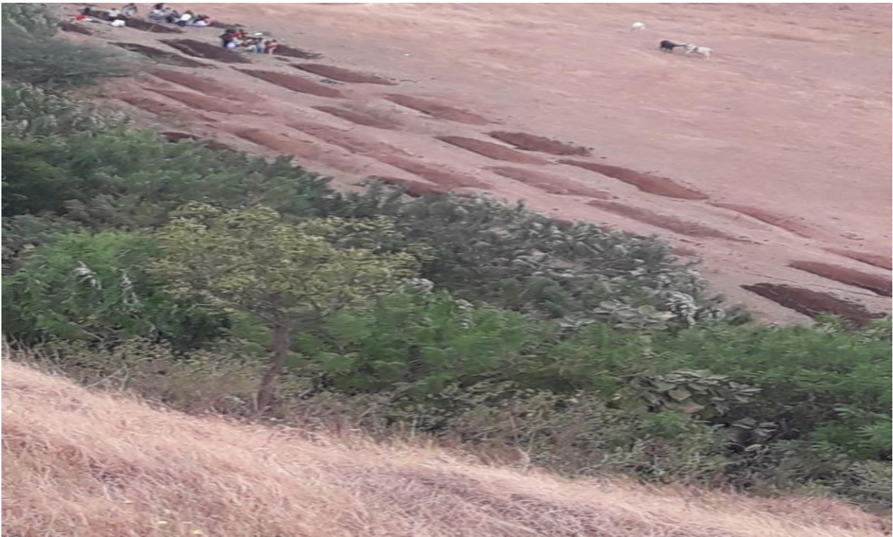
Excavated premises of CCT at NSS camp at Dari
