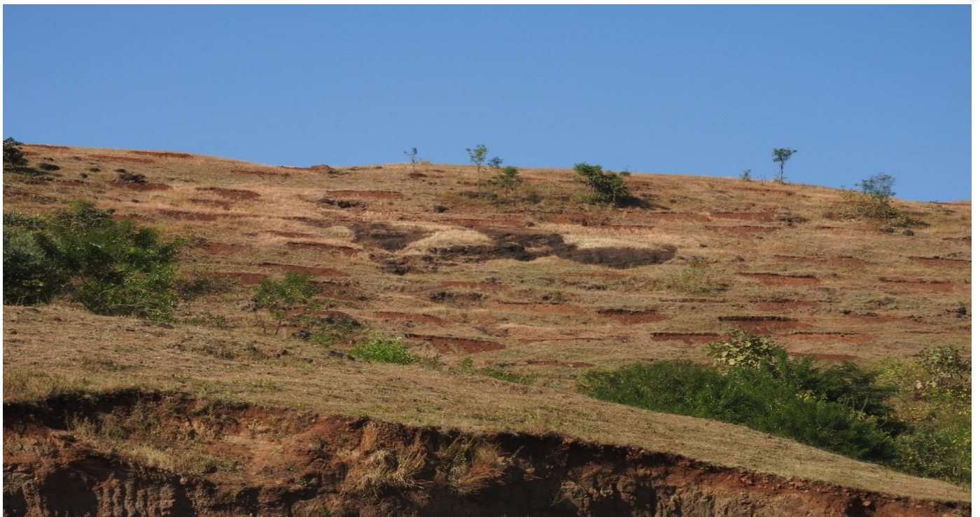
Excavated premises of CCT at NSS camp at Dari
