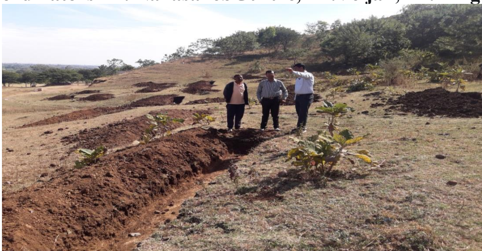
While inspecting the work of the labor camp at Dari, NSS Nashik District Coordinator Prof. Ravindra Ahire, Dr.DattatrayaVeljali, Dr.Gorakshanath Pingale Volunteers digging Continuous Contour Trenches (CCT) on the hill at Dari
